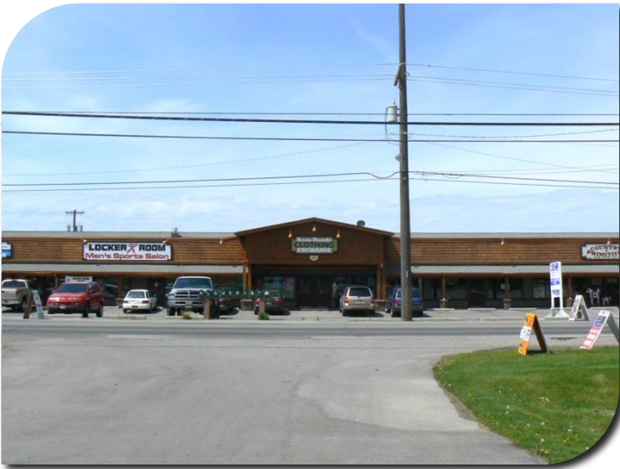
View looking South at Main Strip & Back Building
